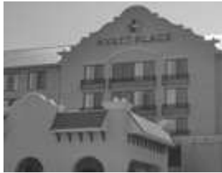
Hyatt Place Fort Worth Historic Stockyards
