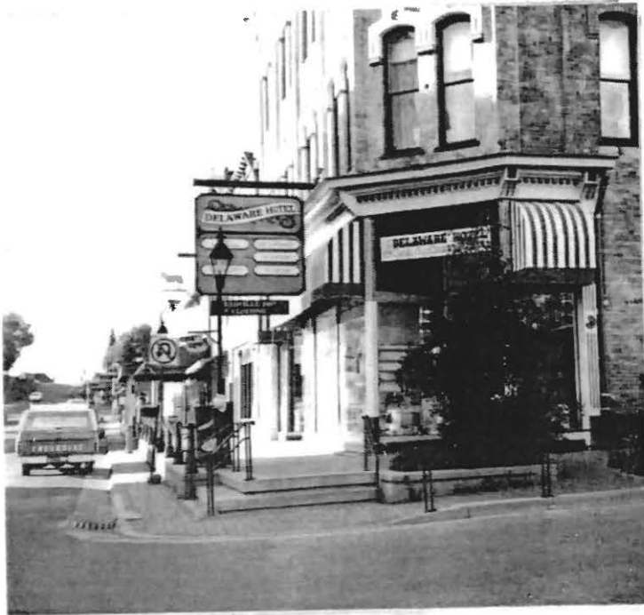
The Delaware Hotel located on 700 Harrison Street in downtown Leadville.
