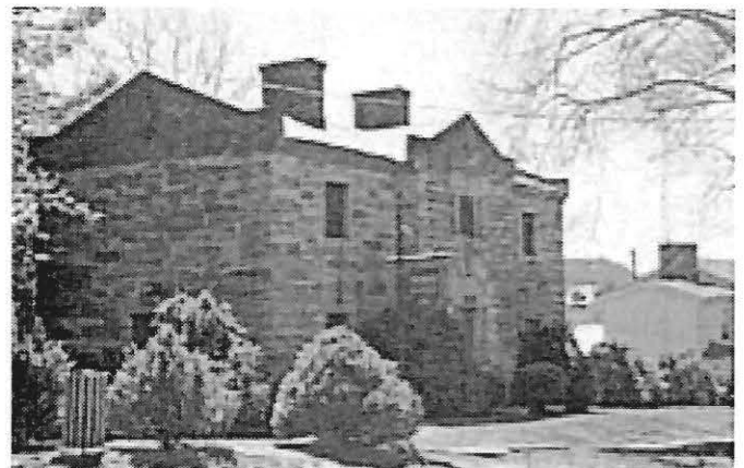
The Fluvanna County Courthouse (top); the former Fluvanna County Jail (above) in Palmyra houses the county historical association.
